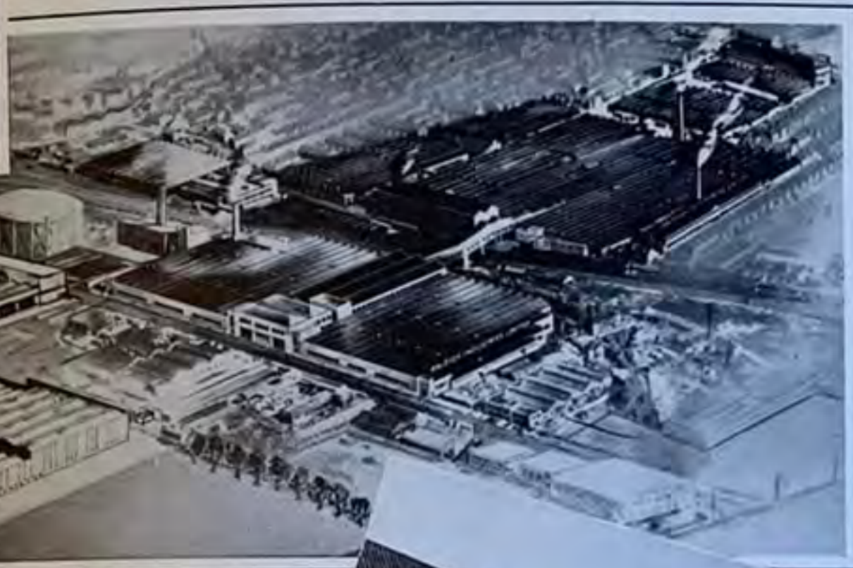
The new factory appears in the centre foreground
