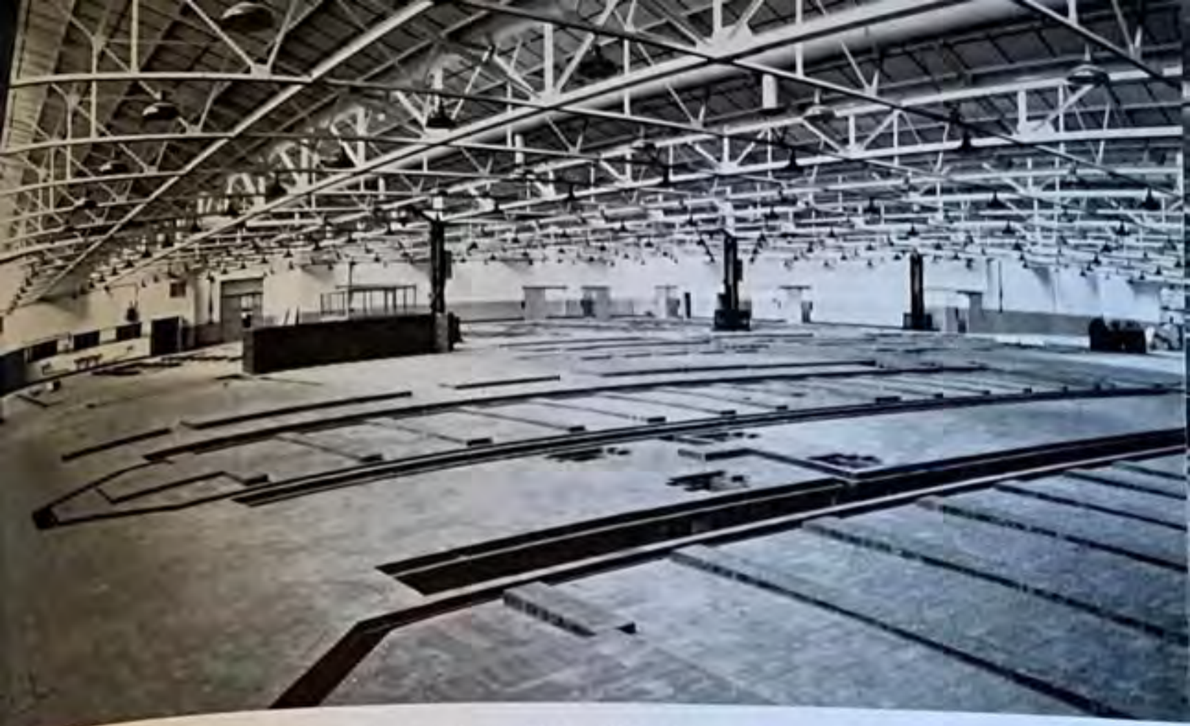
A view of the vast plating shop which will be fully automatic on completion
